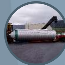
Tanks, silos, vessels
